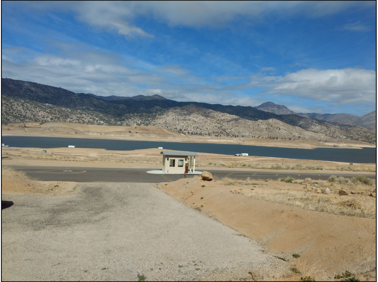
Figure A-15. Photo of the Auxiliary Dam Recreation Area location (Alternative 6), facing northwest.
