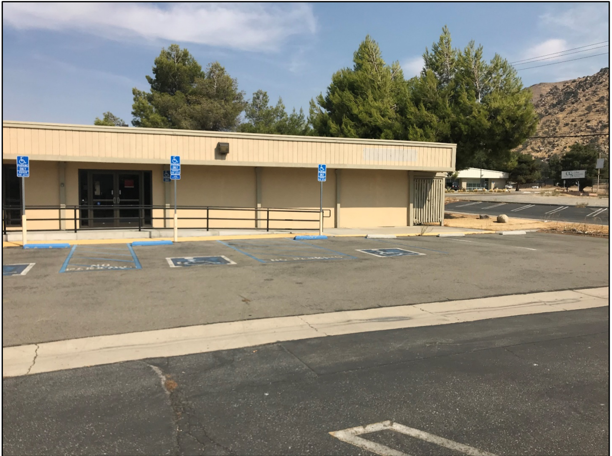
Figure A-6. Photo of the Bank of America building (Alternative 3), facing the south side (taken in 2019).
