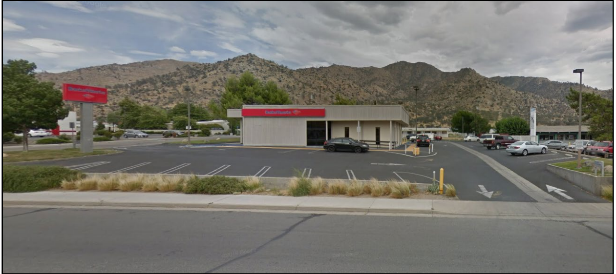
Figure A-5. Photo of the former Bank of America building (Alternative 3), facing the west side with foothills shown in the background (taken in 2015). ©2021 Google
